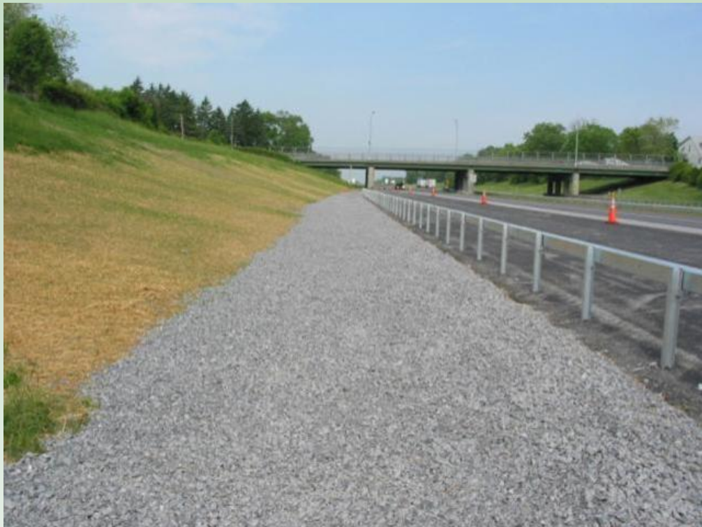
NYSTA Infiltration Trench (Albany Div; Exit 23)
