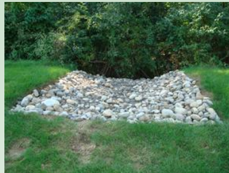
Latham Business Park Infiltration Basin
