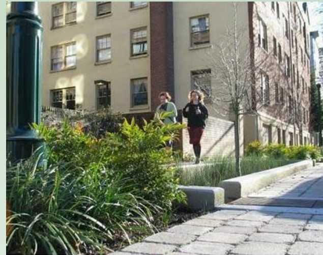
Stormwater Planter - Portland
